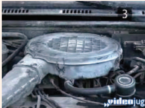
Fig : Cleaning of air filter housing
